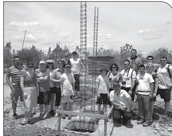
This team of SchoolBOX volunteers took a quick photo break from digging holes and building the rebar for foundation posts. You are invited to volunteer to help build another school in Nicaragua this coming November!
